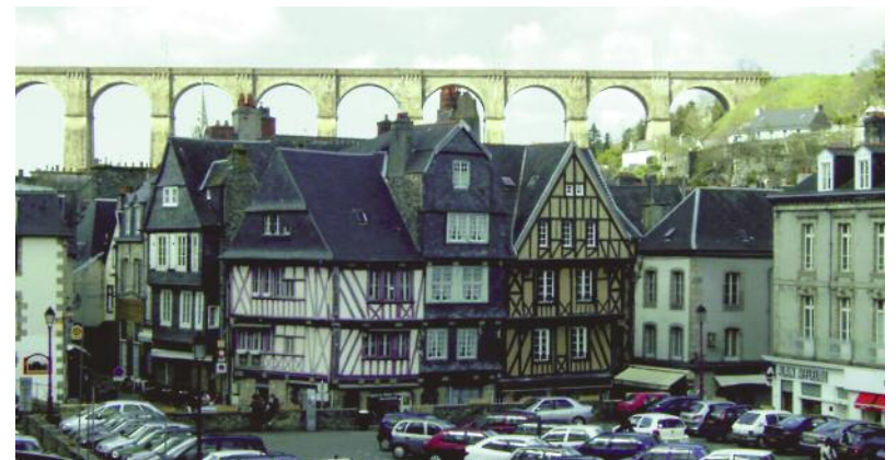
Half-timbered houses on the Market Place
